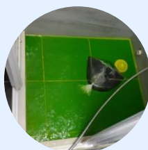
Ponding test for floor slabs
