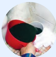
Colour water test for drainage pipes
