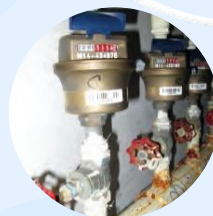
Test for water supply pipes
